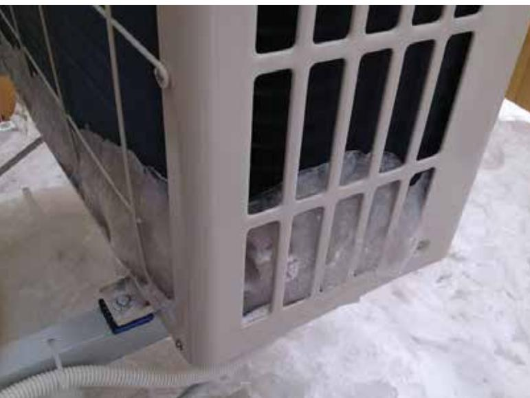
Without the right technology, condense freezes to the bottom of the unit and reduces its efficiency and heating output.
